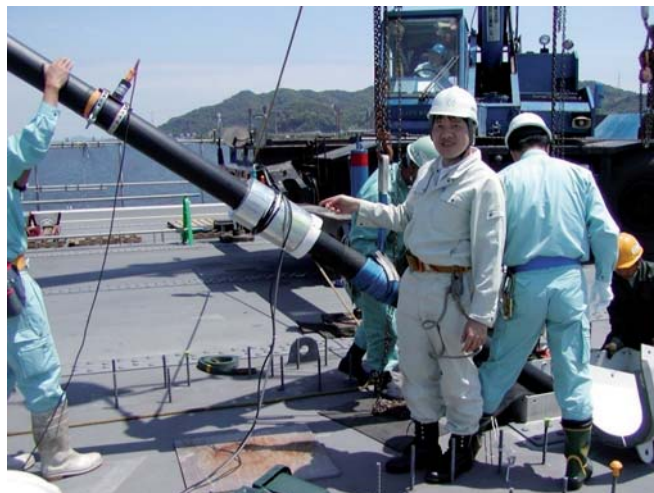
Obr. 2 Delený EM snímač, dodatočne navinutý na záves mosta Ashidagawa, Japonsko; spolupráca s firmou Keisoku Research Consultants, Hiroshima, rok 2002 Fig. 2 Divided EM sensor, additionally wound on a cable stay system of the Ashidagawa bridge, Japan; collaboration with Keisoku Research Consultants, Hiroshima, 2002
